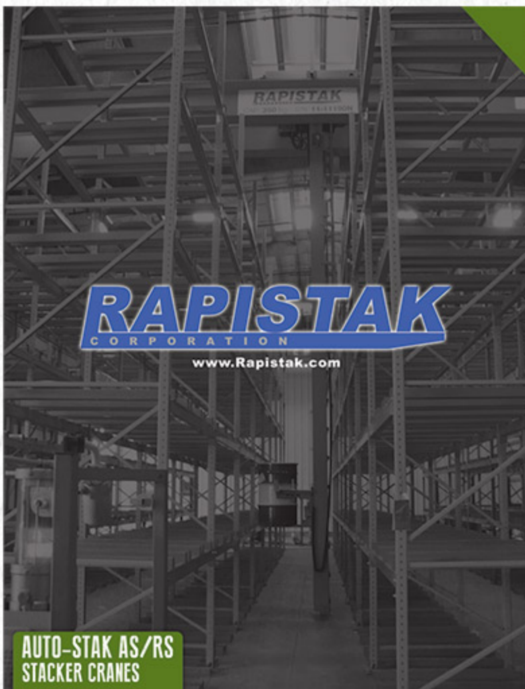
Automated Management Systems
